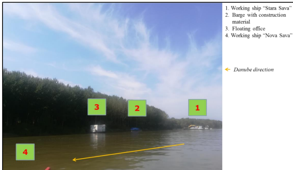
Figure 1 Display of construction sites and auxiliary objects within the Futog critical sector (Futog 2 subsector)
