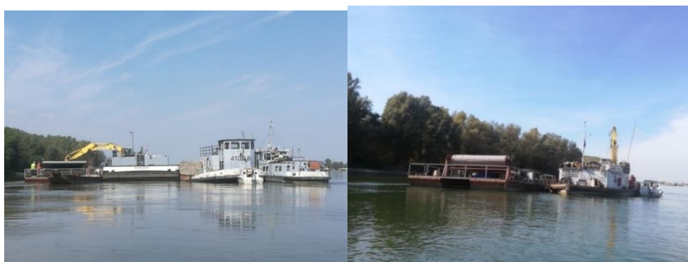
Figure 2 Display of construction sites and working ships "Stara Sava" (left) and "Nova Sava" (right) – upstream view
